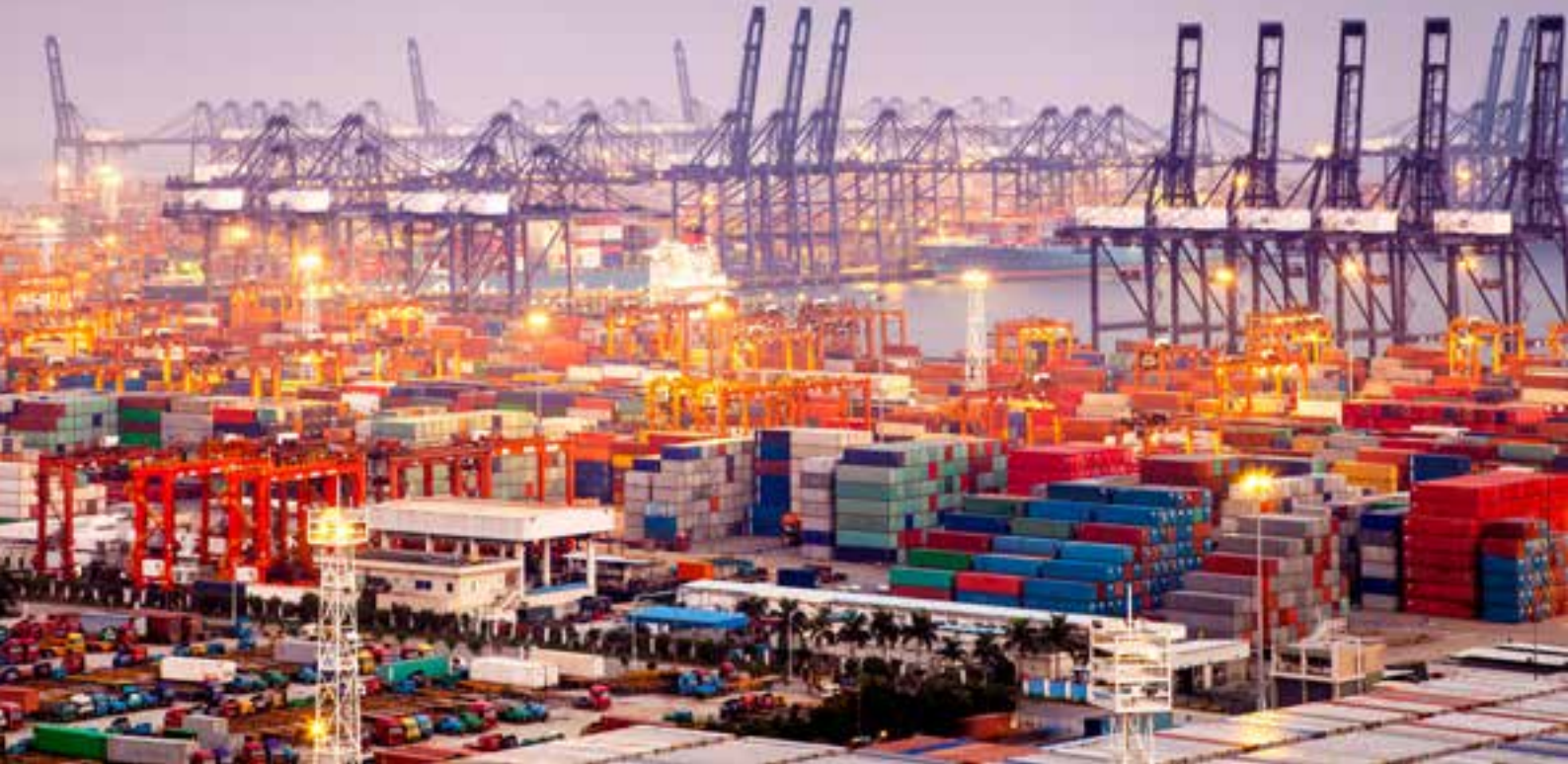
Asia's flow of goods continues to generate demand for material handling solutions.
